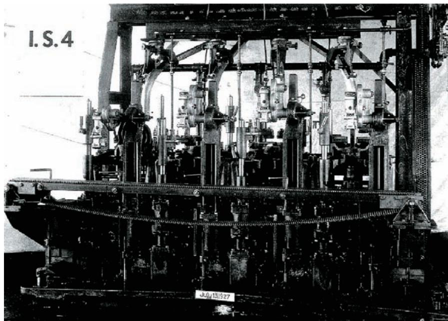
Fig 1. 1927: The first commercial 4 section IS machine.
