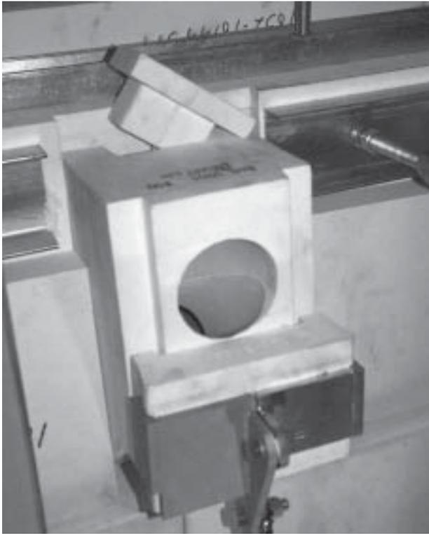
**Figure 2.** Cleanable damper/flue block
